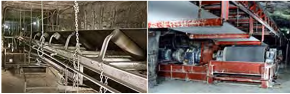
Figure 21-1. Typical Underground Conveyor Installations (from Joy 2010a)
